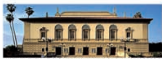
THE PASADENA CIVIC AUDITORIUM
