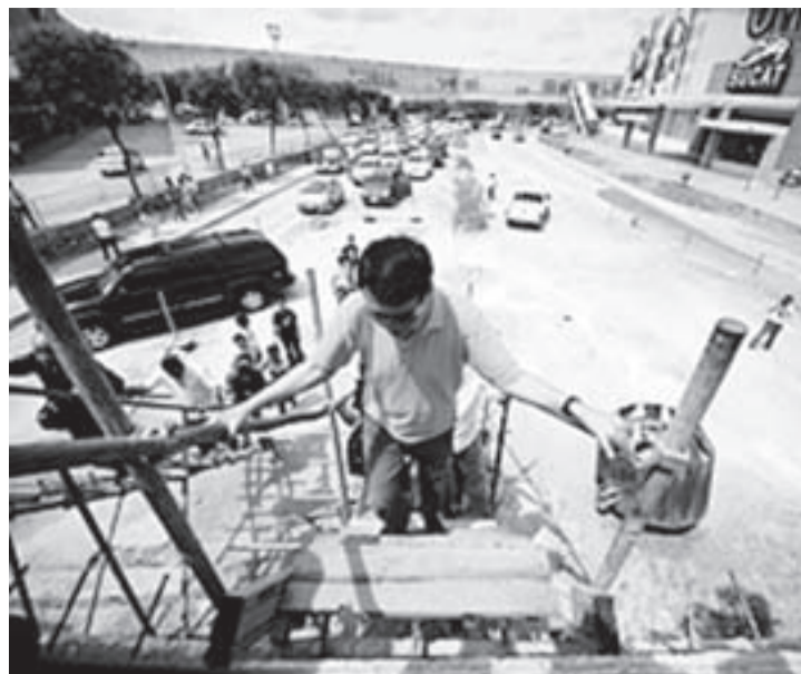
Sen. Manuel Villar Jr. inspects a portion of the C-5 road extension project in Sucat, Parañaque City last May 21. Philstar Photo by Manny Marcelo
